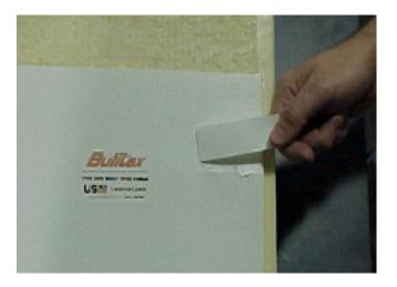
3. Position the repair patch over the tear.
